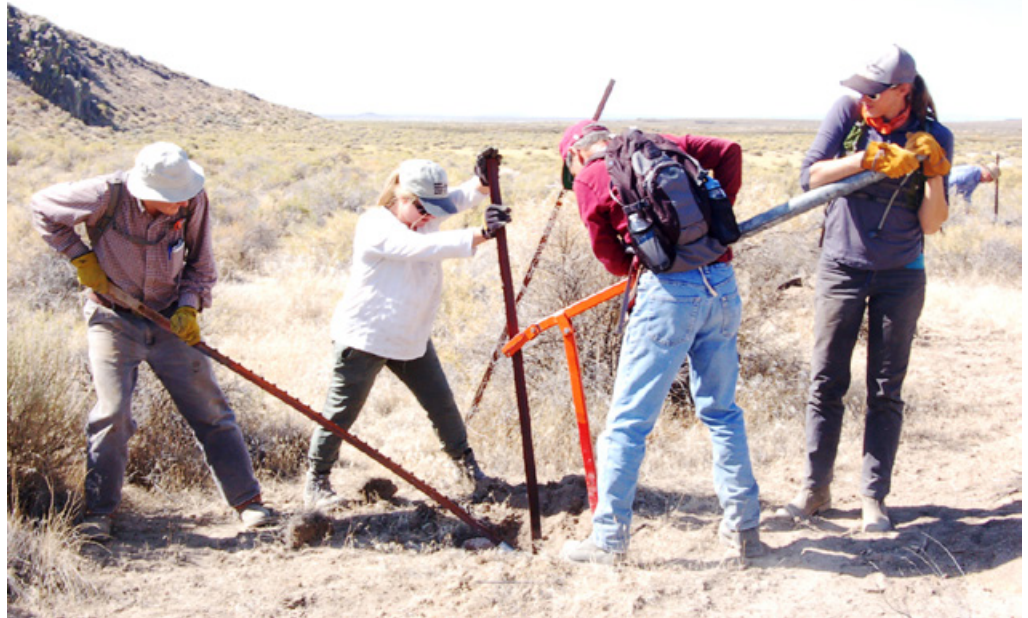
In the Malheur National Wildlife Refuge, alkali soils interact with rusting steel to create a sort of concrete block beneath each fence post, making already tough work into an even more arduous task. Photo: Lisa Foster
