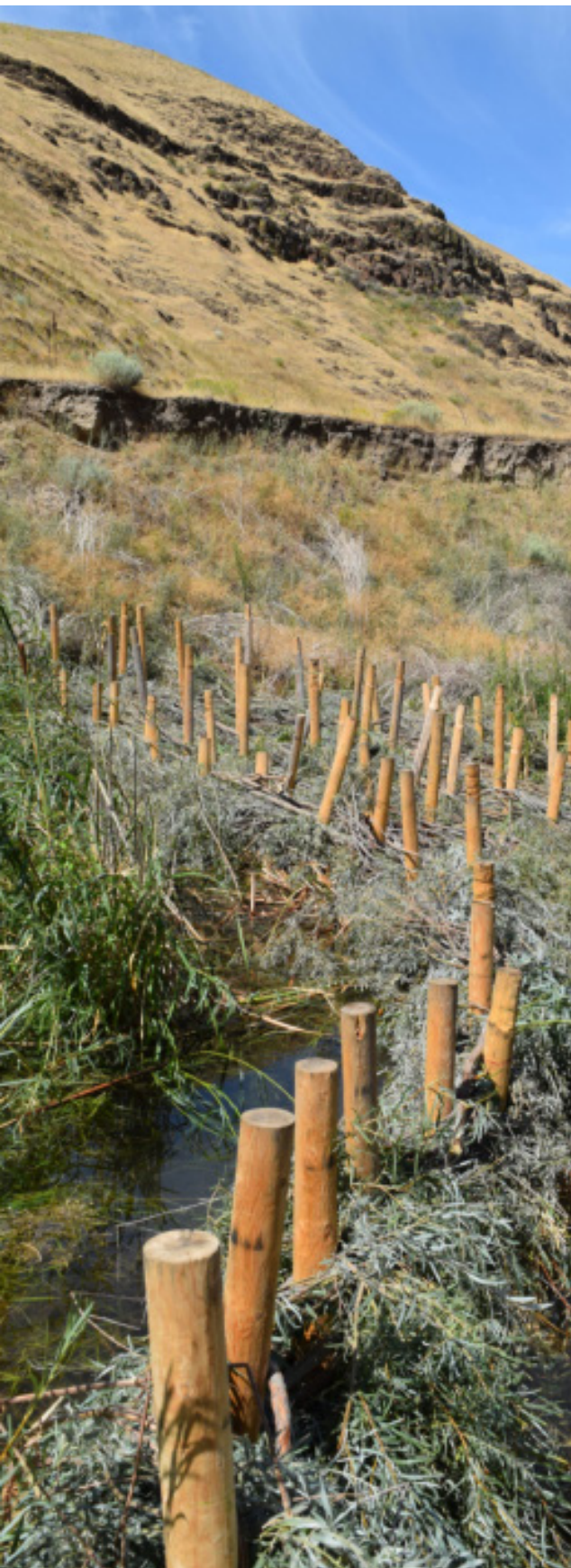
ONDA volunteers have installed dozens of beaver dam analogs in Hay Creek. Photo: Maria Johnson
