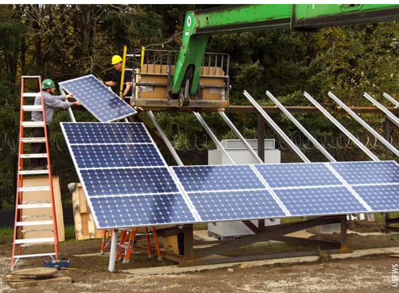
Solar panels under construction.
